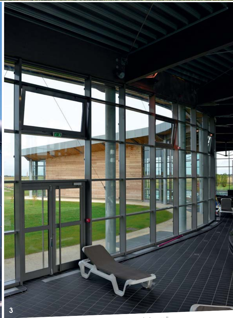
1 Espace® 50TH openable and fixed windows, Comète® 50TH fast-fitting doors - 2 Espace® 50TH windows in Univers® 54 curtain wall 3 Espace® 50TH bottom-hung window, Comète® 50TH fast-fitting door
