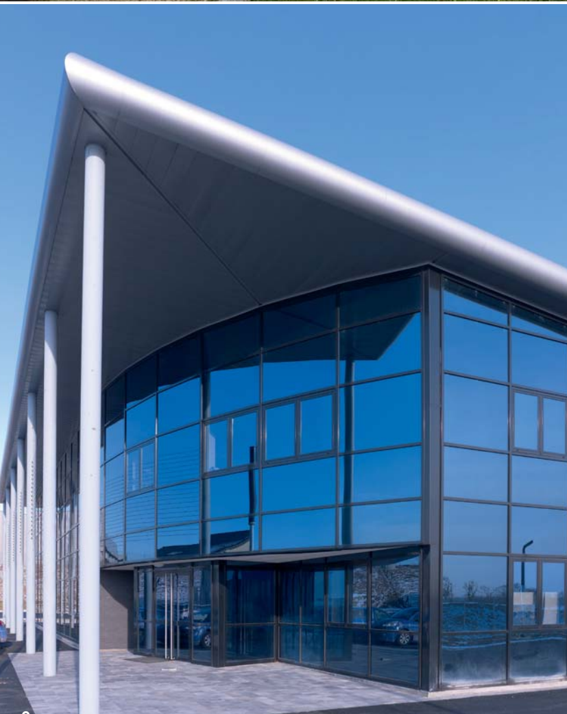
1 Espace® 50TH openable and fixed windows, Comète® 50TH fast-fitting doors - 2 Espace® 50TH windows in Univers® 54 curtain wall 3 Espace® 50TH bottom-hung window, Comète® 50TH fast-fitting door
